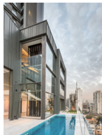
Project in Lebanon
